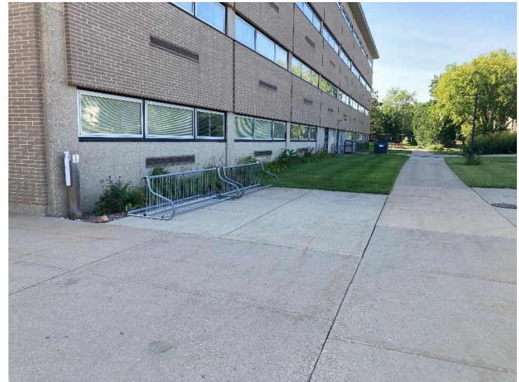
Heide Hall – West side
