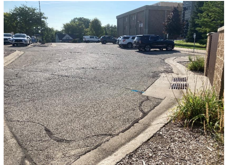
Looking east across the north face of Winther Hall
