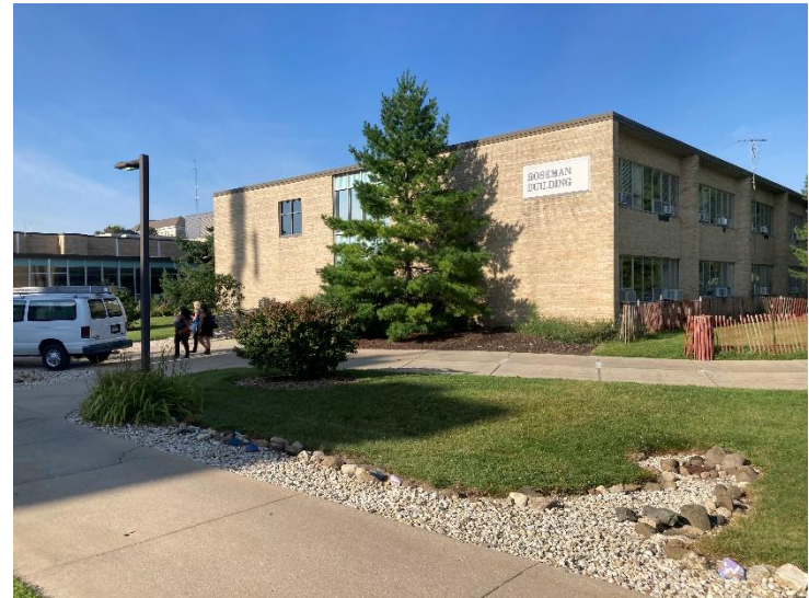
Roseman Building (east side)
